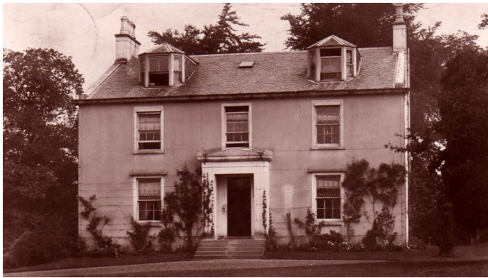
Strathblane Manse, completed in 1828
